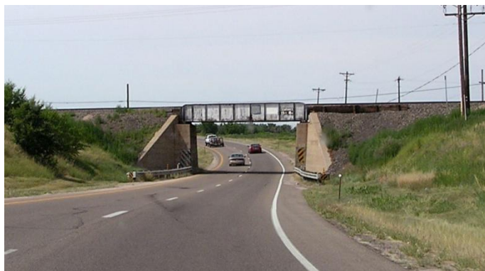
Figure 4-28. BNSF Railway Crossing of US 50—La Junta
