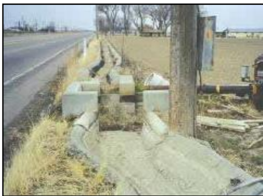
Figure 4-81. Examples of Inadequate Clear Zones on US 50
