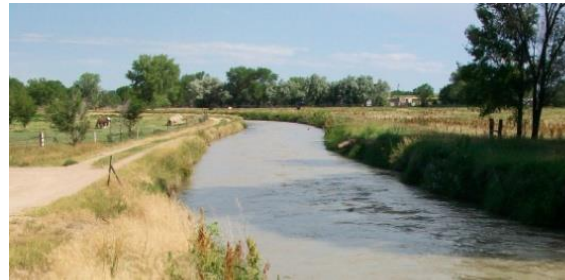
Figure 4-60. Catlin Canal (View from US 50)—Otero County
