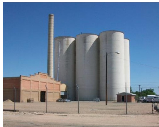
Figure 4-9. Agricultural Product Storage Facility—Rocky Ford
