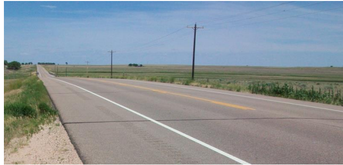
Two-Lane Segment of US 50 (Bent County)
