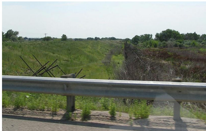
Figure 4-29. Arkansas River Levee—Las Animas
