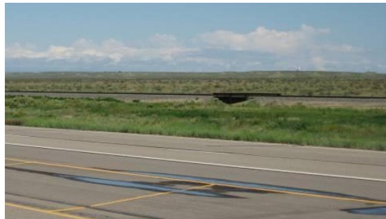
Figure 4-63. Railroad Track Adjacent to US 50—Pueblo
