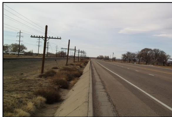
Figure 4-81. Examples of Inadequate Clear Zones on US 50
