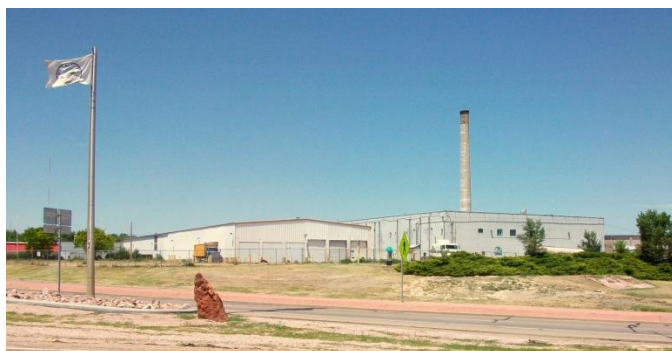
Figure 4-55. Bay Valley Foods Plant—La Junta
